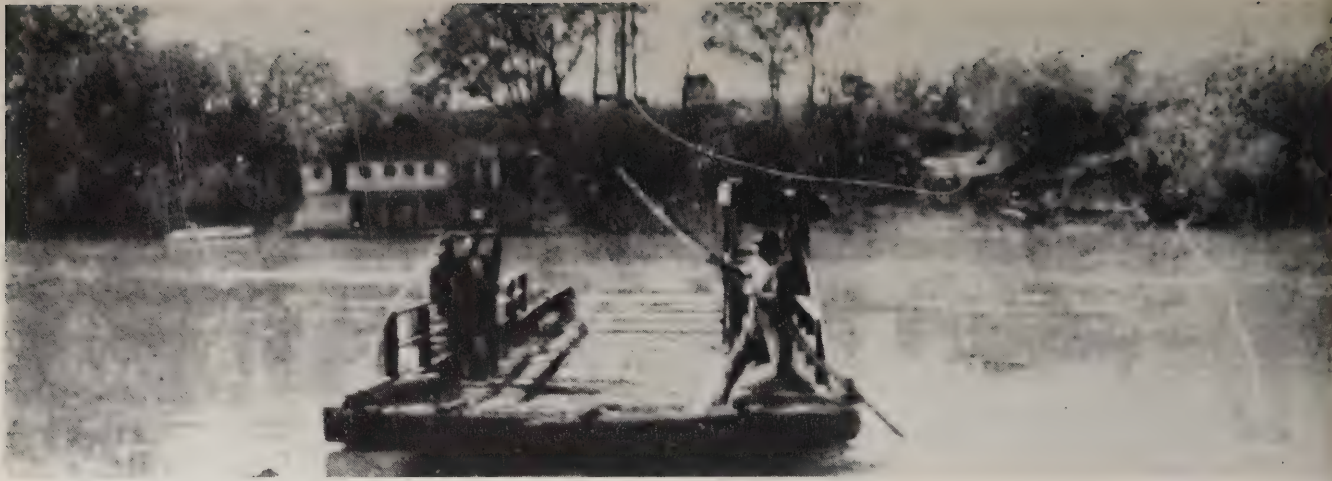
This ferry was run in both directions by the current of the river.
